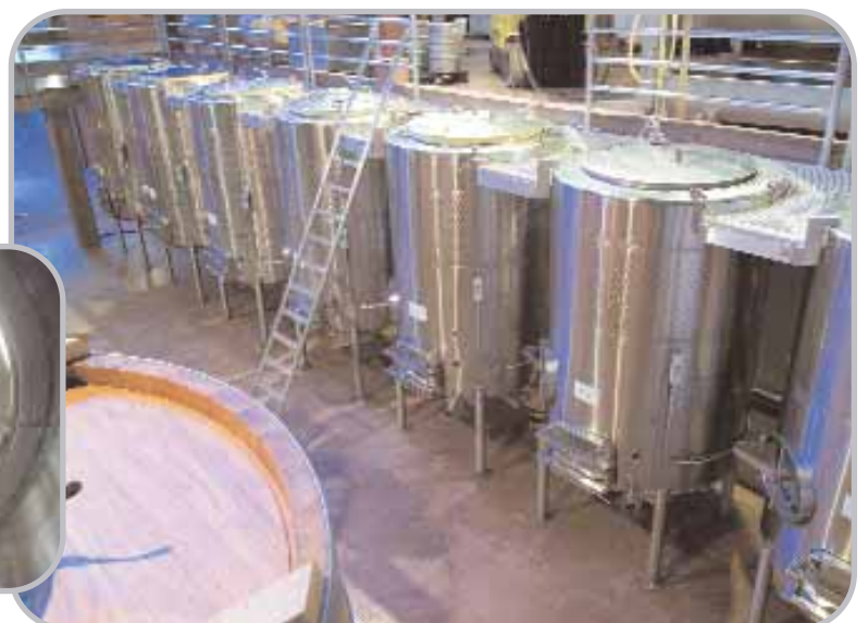
Convertible Fermentation Tanks, installed.
