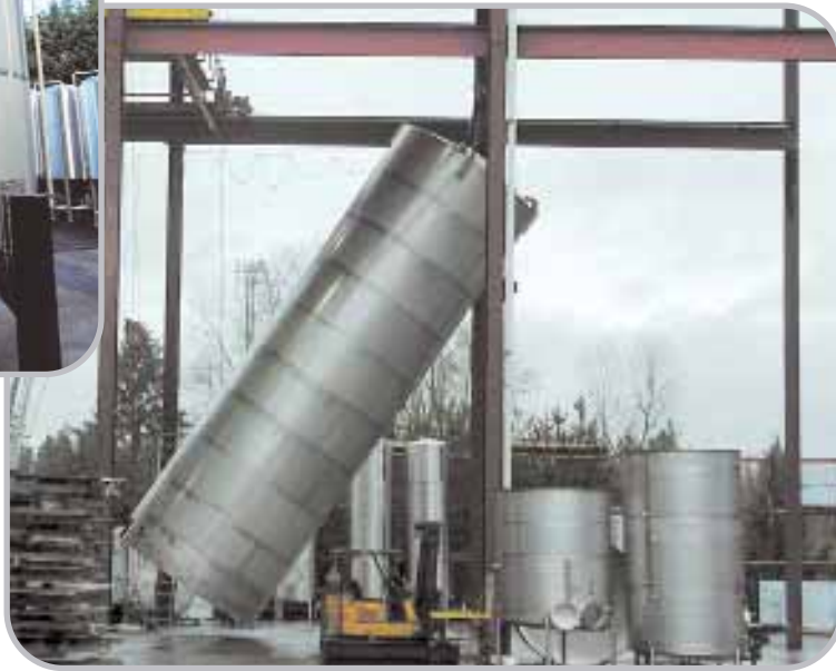
Tip-up Formula Clearance (C) needed for tip up: C = \sqrt{A^2 + B^2}
