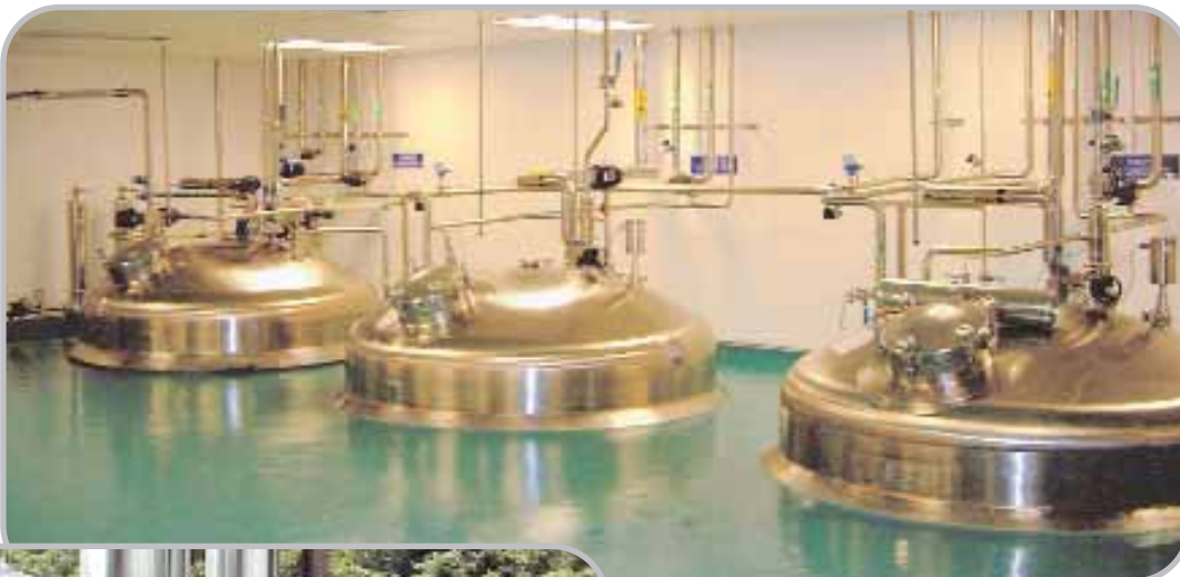
IV Batch Production Line Vessel—installation.
